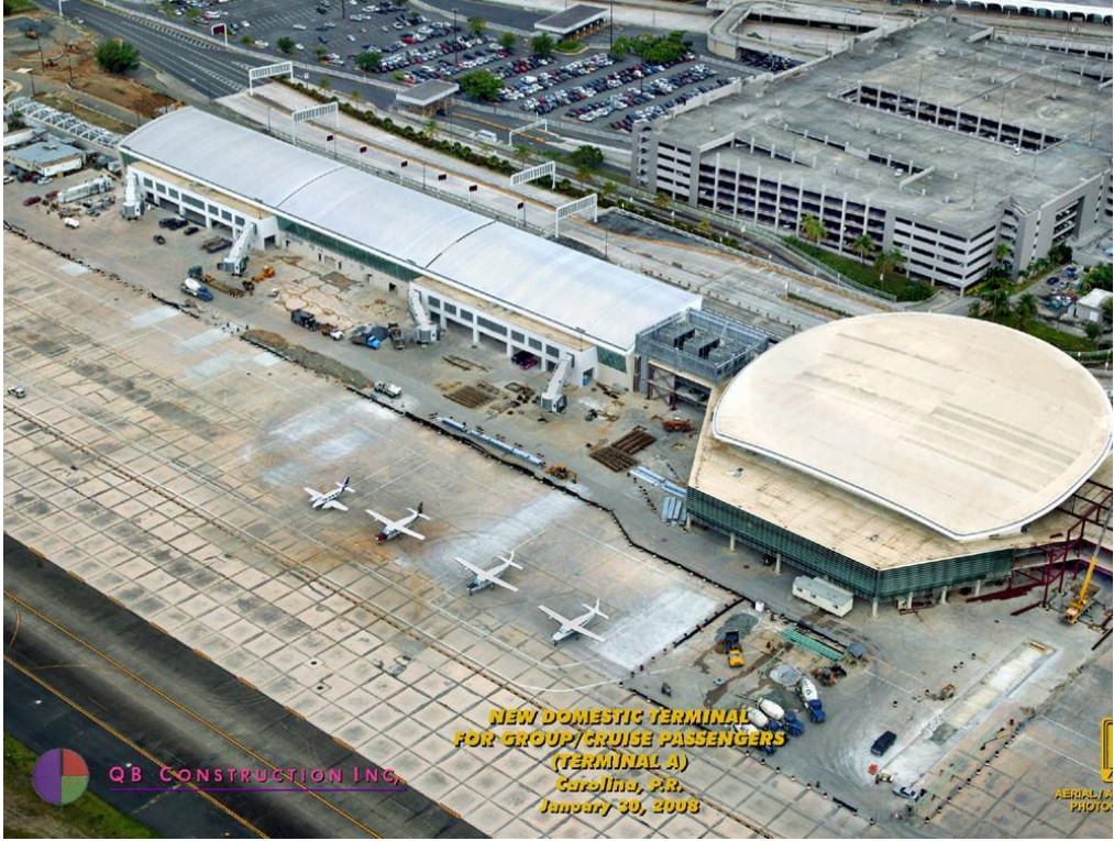
apron and new domestic terminal aeral view (d) ©QB Construction and AAPA Aerial / Architectural Photography, Inc.
